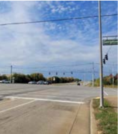
Existing Overhead Utility at the Intersection
