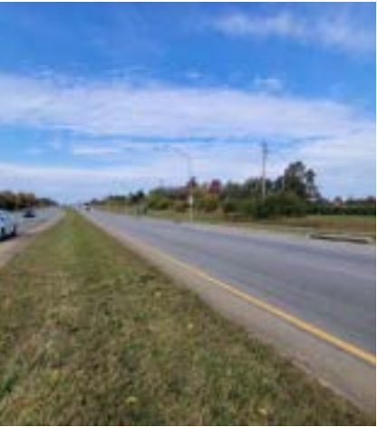
Existing Bus stop and Median
